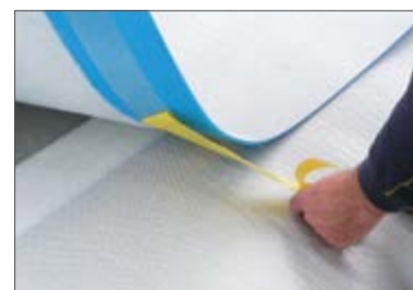
(2) Remove the protective yellow band to fix the lateral layer
