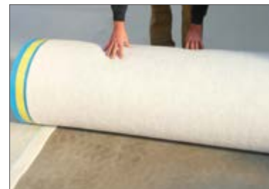
(1) Unroll the underlay with the overlap over the lateral roll
