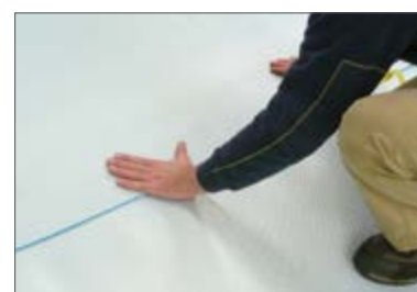
(3) Stick correctly the two layers together
