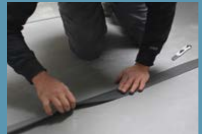
Insure the tightness with the Stickelfoam 25/70
