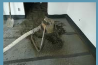
Make a ± 8 cm thick reinforced screed on the Bi+20
