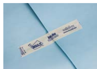
(2) Keep the overlap maintained with the adhesive provided
