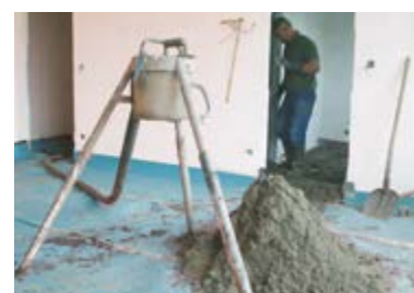
(4) Make a \geq 5 cm thick screed up the insulit 4+2
