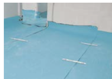
(3) Place the underlay alongside the wall ( \pm 15 cm)
